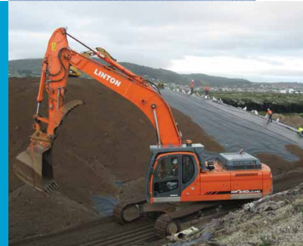
Waste carbon pile covered in plastic and pea gravel at the NZAS landfill
